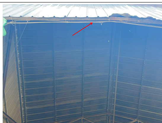
入料棚门口喷淋设施
