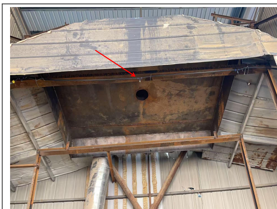
入料棚内喷淋设施
