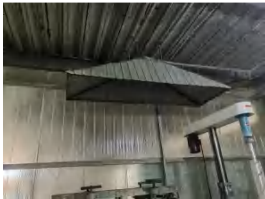
粉状物料投料工序集气罩
