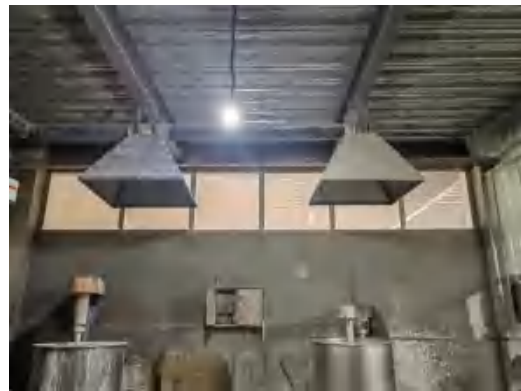
粉状物料投料工序集气罩
