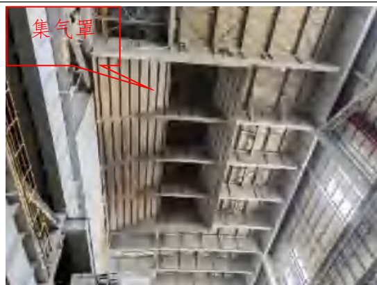
炼钢车间顶部集气罩
